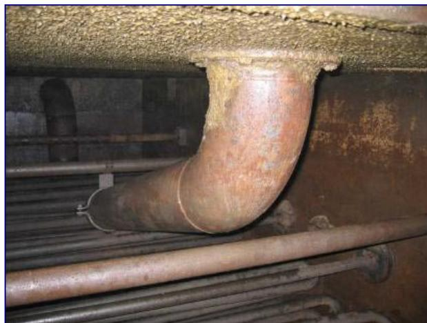
*Photo 3: Lub oil tank (25 m<sup>3</sup>) after cleaning.*
