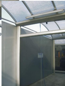
Deposit on stainless steel parts of car wash stations
