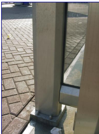
Deposit (upper surfaces) and after treatment with Stainless Steel Cleaner (lower surfaces)
