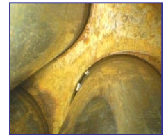
Internal inspection of a heat exchanger
