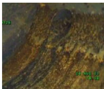
Fig. 4: Surface prior to the cleaning
