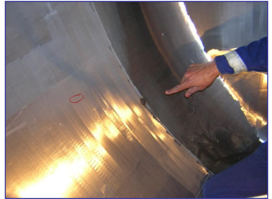
Defects before and after filling by TIG welding
