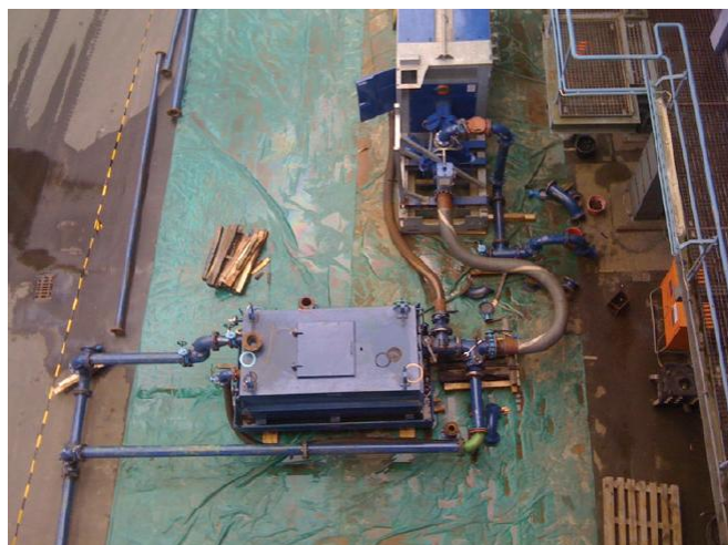
Pre-commission cleaning with Demclean 94®
