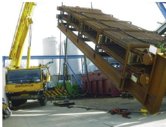
Pre-commission cleaning of a heat exchanger using VPX One Step®
