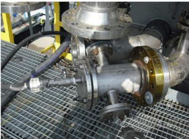
Receiver/launcher of the pigs
