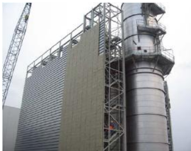
Photo 1: Unit 4 of the Flevo power under construction
