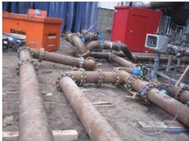
Photo 3: Temporary lines for chemical cleaning (DN250)
