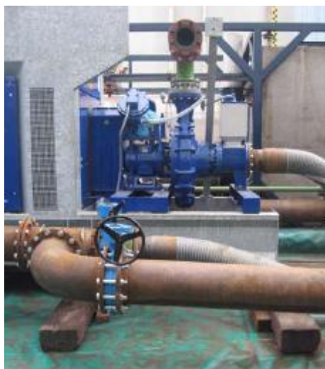
Photo 2: erection of the cleaning equipment (850 m 3 /h diesel driven pump)
