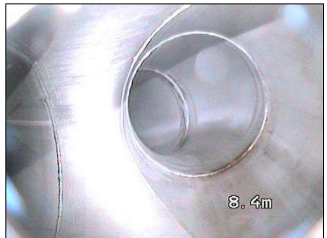
Line 4 (after treatment) – Pickling successful, some evidence of trapped air pockets caused by vessel trim
