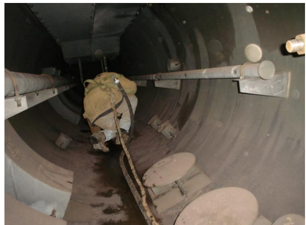
Figure 2: Steam drum after pickling and passivation
