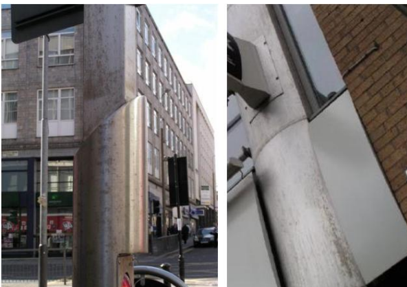
Photo above and below: Corrosion on public stainless steel objects
