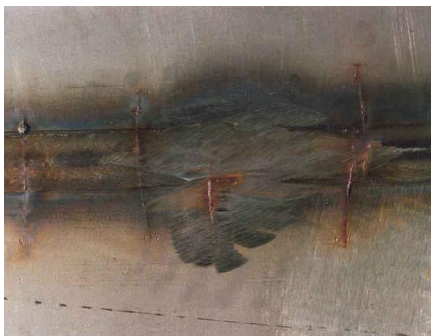
Photo 1 Cracking in X2CrNiMoN22-5-3 MVC stripping columns
