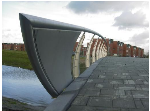
Example of outdoor applications: ceramic blasting of a stainless steel bridge railing
