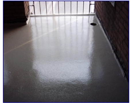
Floor after cleaning and conservation
