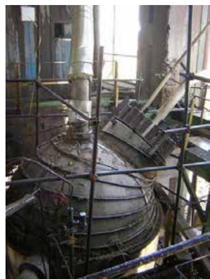
Upper surface of a urea stripper in Iran
