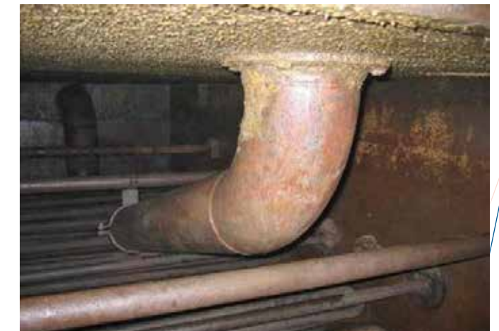
Lub oil tank (25 m 3 ) after cleaning
