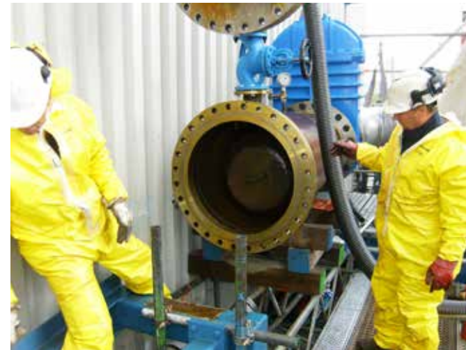
Pig launcher
