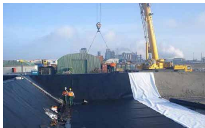
Applying foils using a crane: first the white protective foil, next, the black EPDM foil
