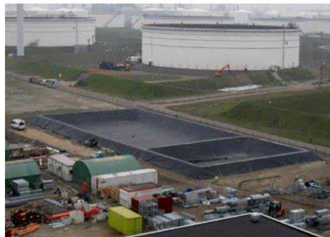
An effluent pit after the earthworks (top) and the final result (bottom)
