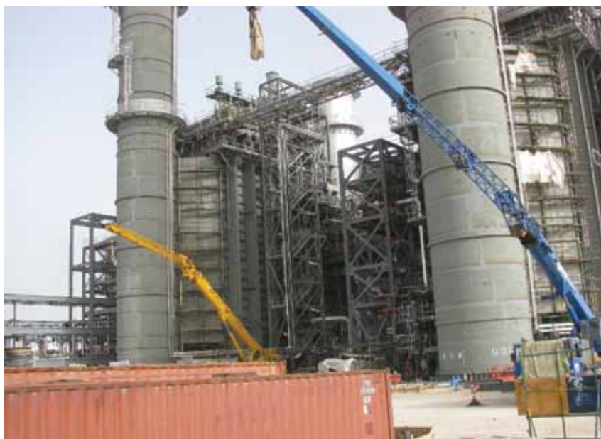
Heat Recovery Steam Generator.
